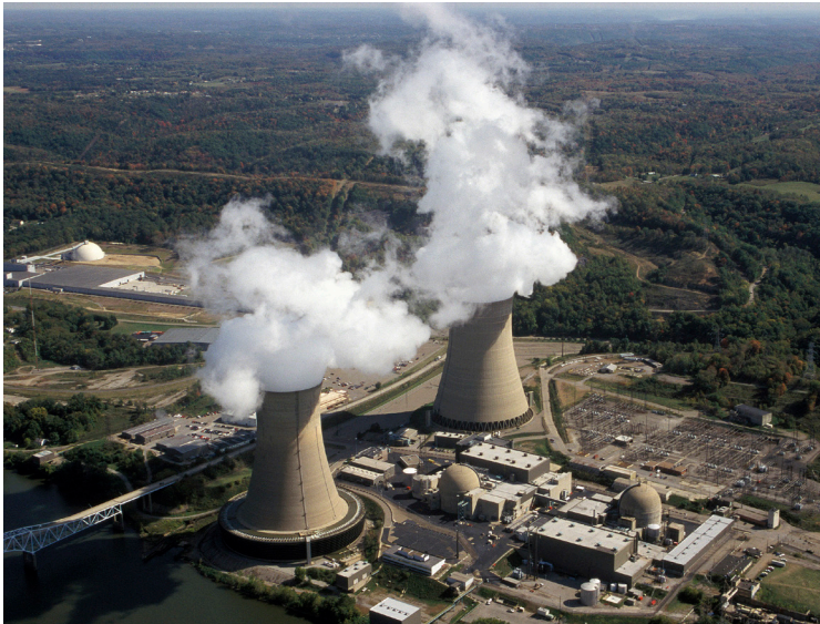
The Beaver Valley Power Station is located on a 453-acre site along the Ohio River in Shippingport, Pa.
