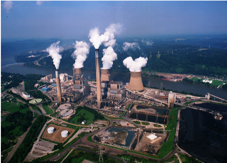
The plant is located in Shippingport, Pennsylvania, along the Ohio River, approximately 25 miles northwest of Pittsburgh. The site covers 473 acres.
